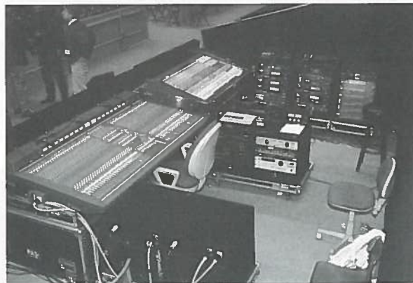
The sound system set-up with a Yamaha PM4000 and Midas XL2 providing the main FOH control.
